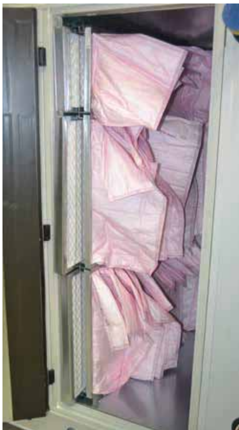
Side withdrawable combined filter (panel + bag)
