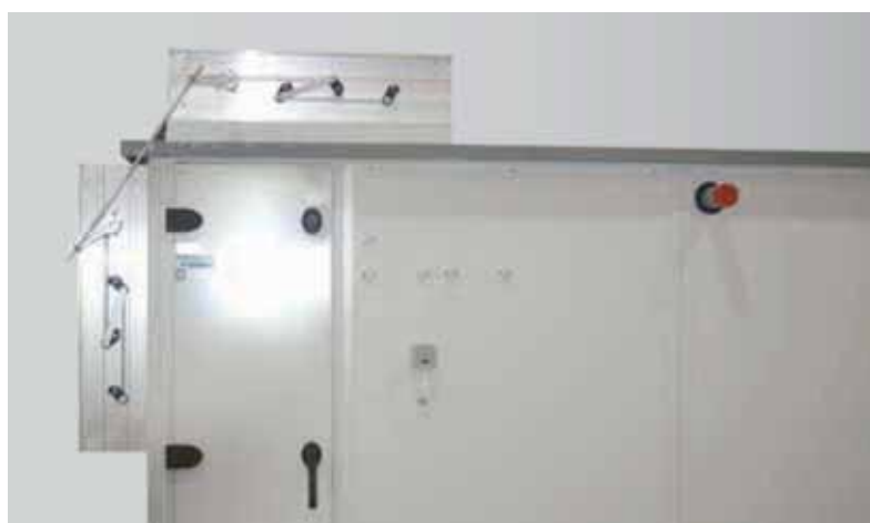
Coupling rod for dampers
