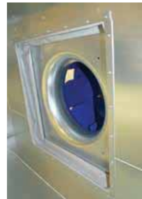
M0 fire class fan flexible connection
