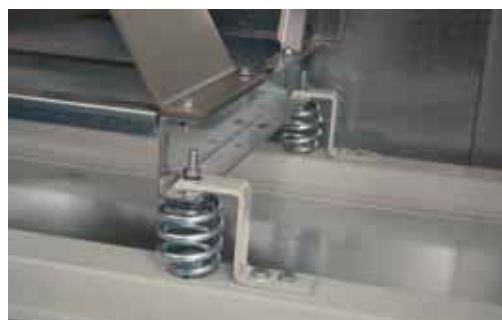
Spring anti vibration mounts
