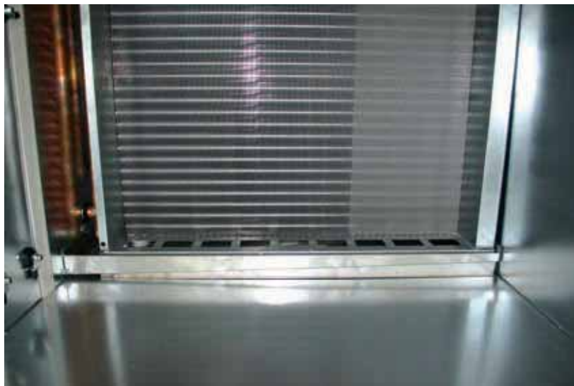
Sloped drain pan
