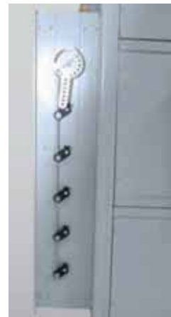
Damper movement mechanism
